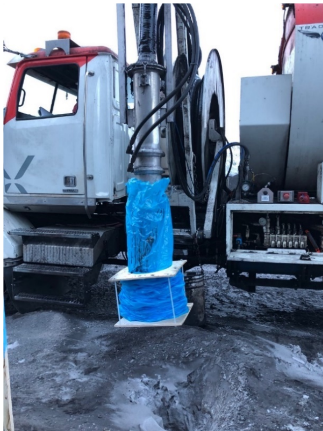
Figure 13. Example of Liner and Emulsion Being Loaded into a Wet Hole. Source: Teck.
